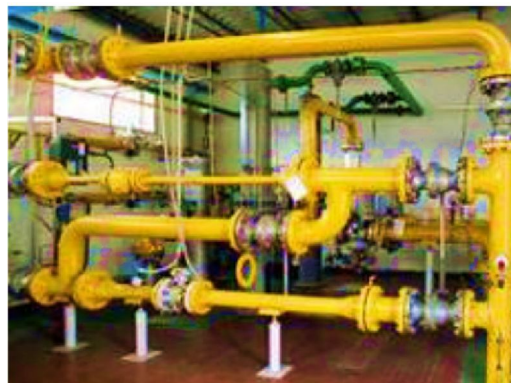
Fig 3: Station for reducing the force of pressure.
