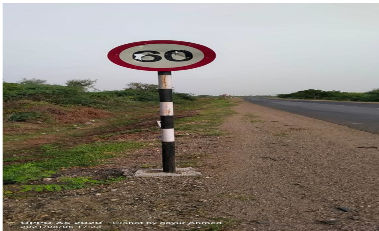
Ch. 26+500 Damaged speed limit sign board
