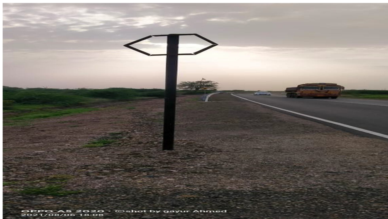
Sign board found damaged at Ch. 7+290
