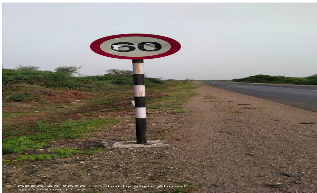
Ch. 26+500 Damaged speed limit sign board
