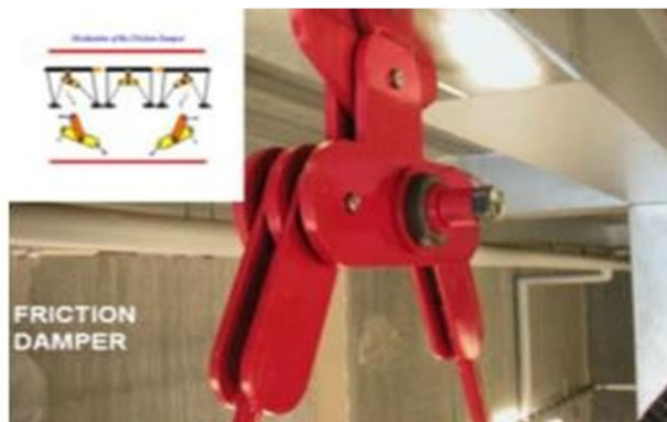
Fig1: Friction Damper
