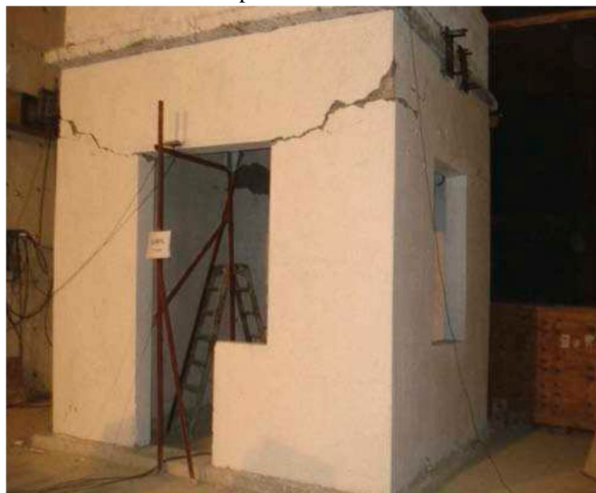
Fig. Final damage pattern for the retrofitted building
