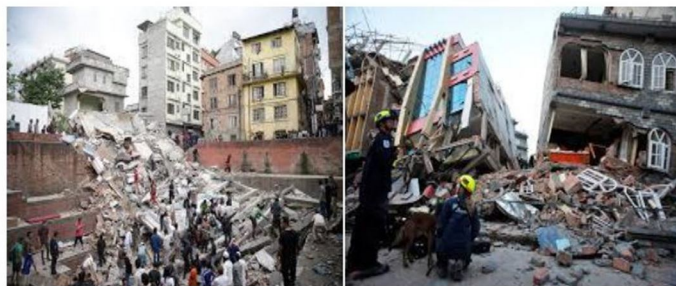
Fig.1.1–Structural devastation from the 2015 Nepal Earthquake (Mw7.8), illustrating the vulnerability of unreinforced and poorly detailed RC construction.
