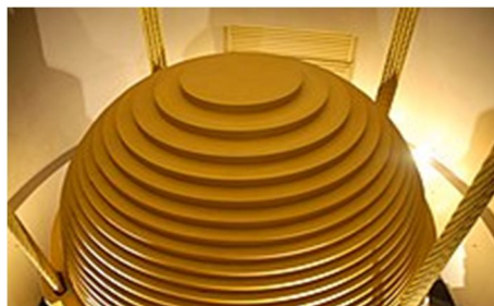
Fig. Tuned mass dampers
