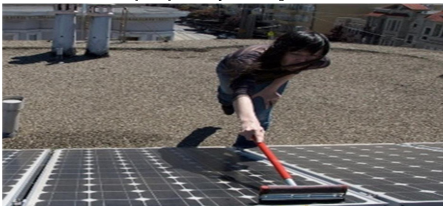
Figure 2 Manual cleaning of Solar Panel
