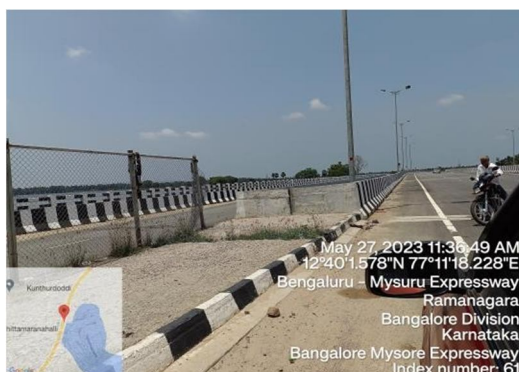
No Advance Warning About Curve/Cheron Marker/Delinator
