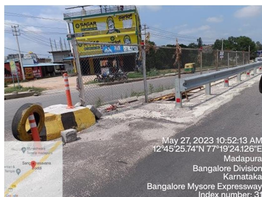
No Dip Sign Board/No Advance Warning
