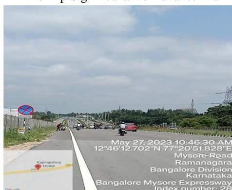
No Dip Sign Board/No Advance Warning
