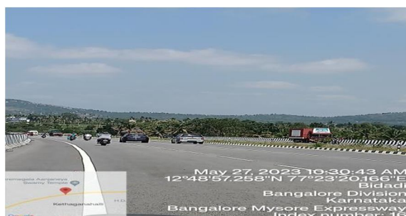
No Advance Warning About Curve/Cheron Marker/Delinataor
