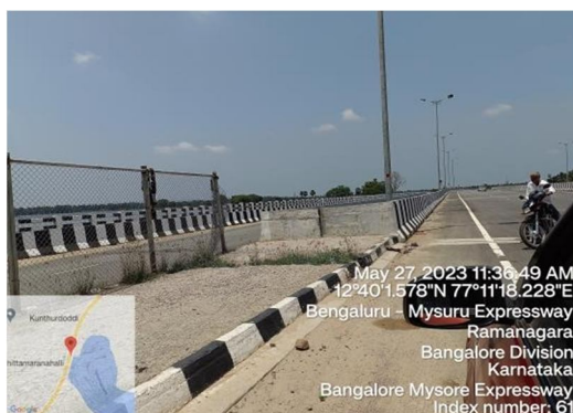
No Advance Warning About Curve/Cheron Marker/Delinataor
