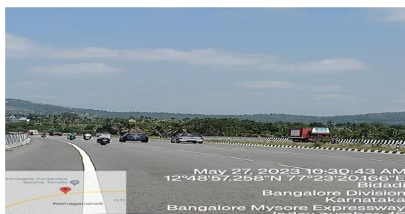
No Advance Warning About Curve/Cheron Marker/Delinator
