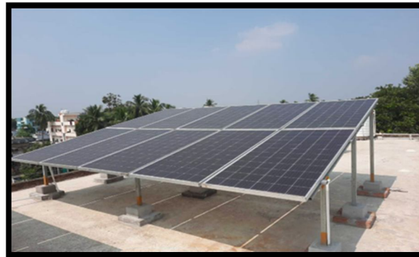
Fig. 10: PV Array pic for 5kWp system
