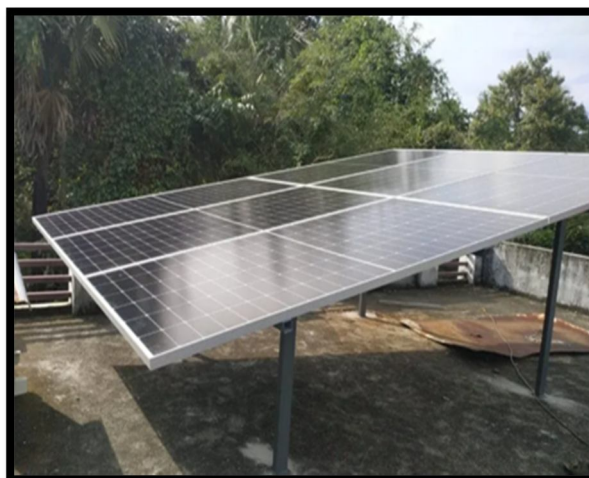
Fig. 7: PV Array pic for 3kWp system
