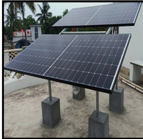
Fig. 4: PV Array pic for 1kWp system
