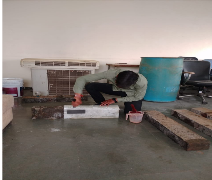
Figure 1. Application of GFRP
