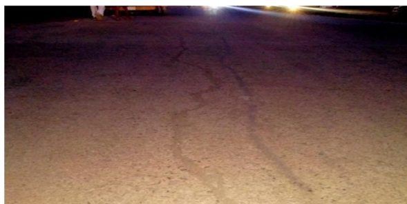
Fig:- Block cracking
