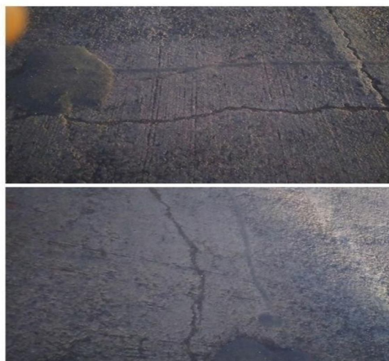
Fig:- Transverse Cracking
