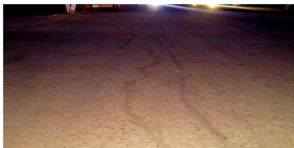
Fig:- Block cracking
