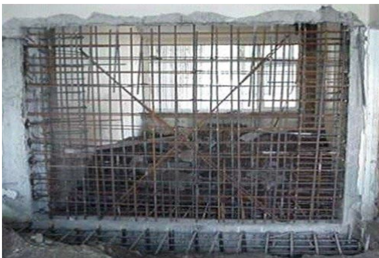
Fig1.1 Additional Shear Wall
