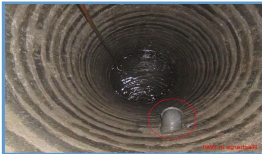
Figure 5 Dug well recharge
