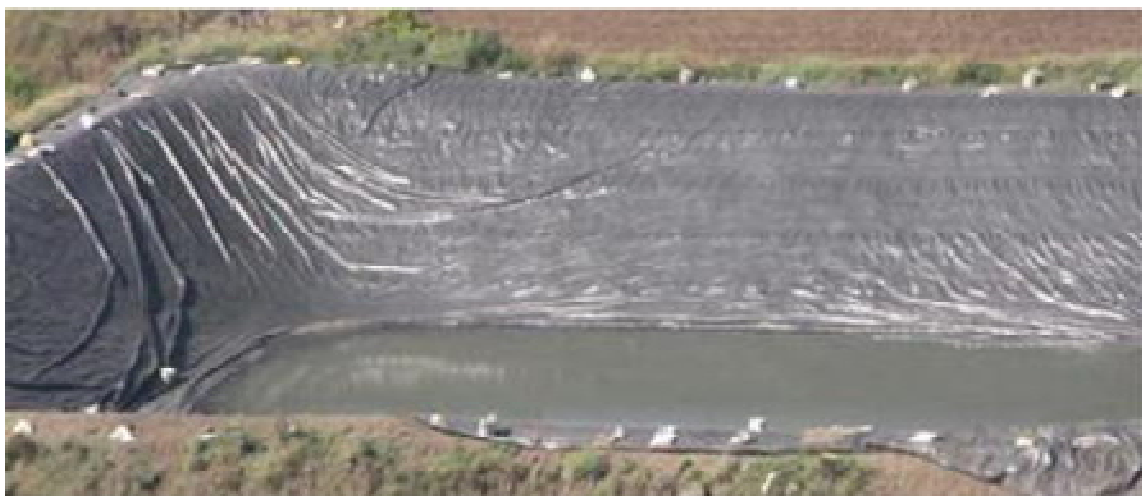
Figure 2 Percolation tank for water storage.
