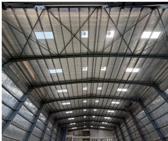
The existing structure views
