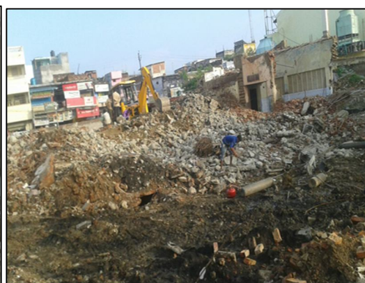
Fig 2 : Demolished aggregates on site
