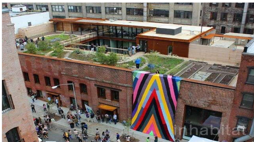
Figure 4—Image shown the façade of Kickstarter Commercial Headquarters (Source: In habitat)
