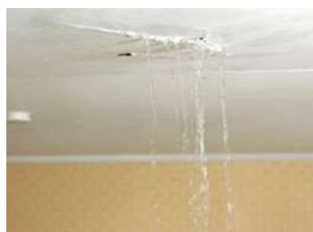
Fig 1: Slab Leakage. Source: www.connectedrestoration.com
