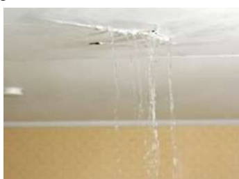
Fig 1: Slab Leakage. Source: www.connectedrestoration.com
