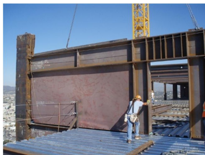
Fig-3: Pictorial representation of SPW
