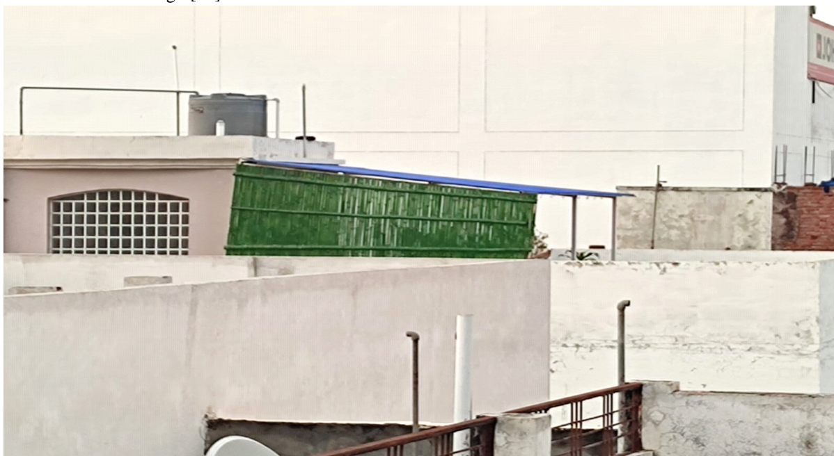
Fig: 3 use of bamboo sticks as a shading
