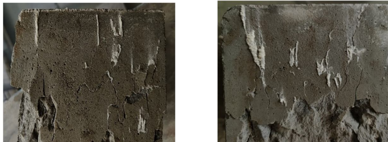
Fig7&8: Filling of cracks in cubes
