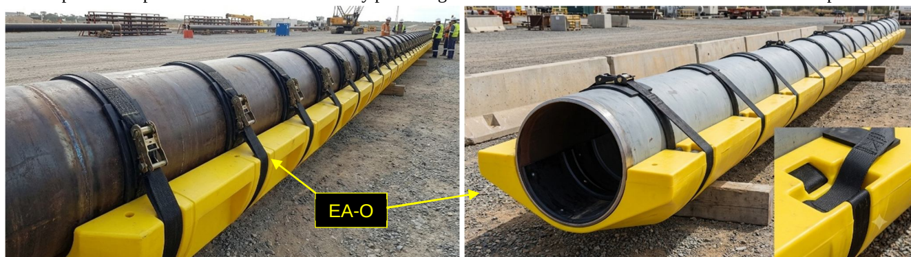
Fig. 13. Examples of Shroud Attachment to Pipeline (Representative Image)
