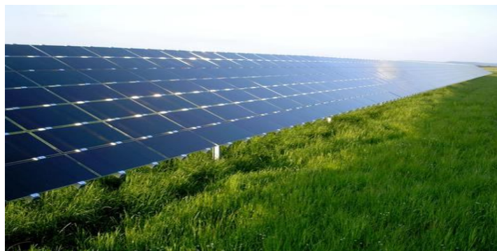
Fig. 2 Glass Substrate based First Solar's CdTe-CdS Solar Panel
