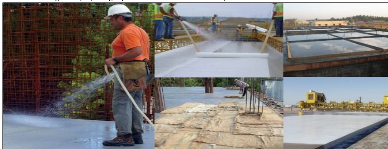
Figure I Different Curing Methods Of Concrete
