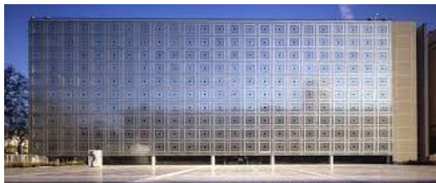
Figure 14. Southern elevation of the Arab World Institute. The developed Mashrabiyya covers the whole façade surface
