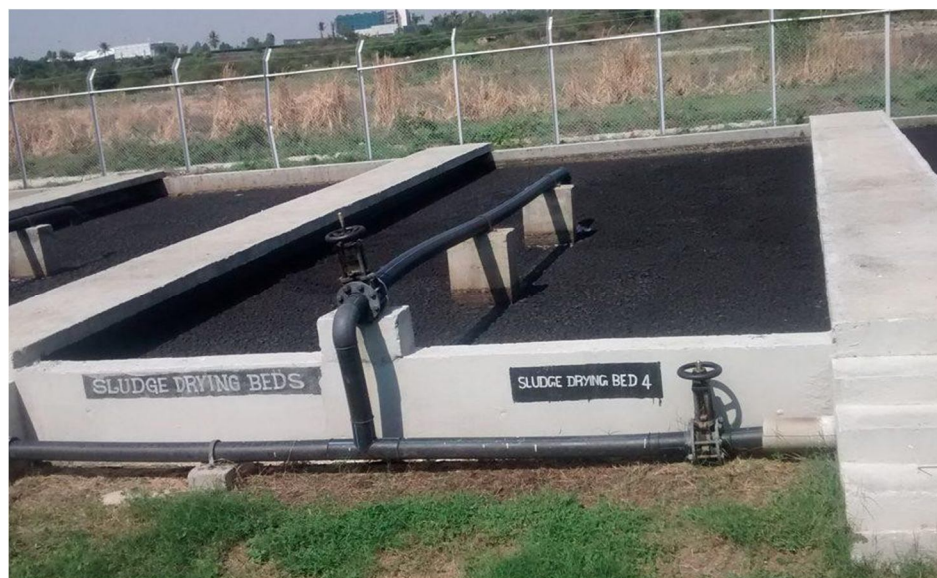
Figure 6: Sludge Management Area
