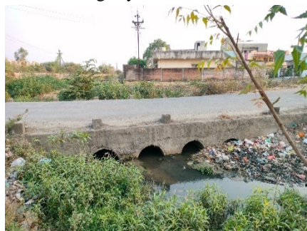
Figure3.1: Existing drain under bridge
