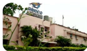
GRIDCO, Bhubaneswar, Odisha
