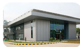
Eco Commercial Building (ECB) Bayer Material Science, Greater Noida, UP
