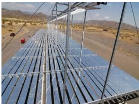
Figure 8 Fresnel Reflector
