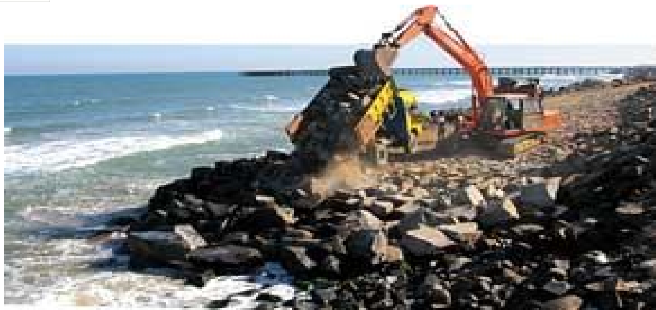
Figure 6: Rubbled Mound Construction At Puducherry Sandy Beach
