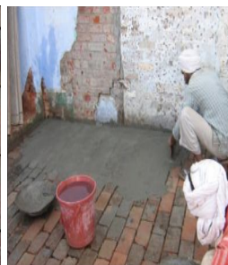
Neat cement slurry
