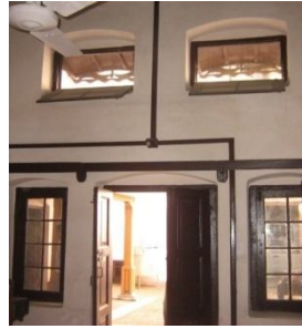
Traditional wiring restored
