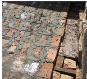
Second layer of brick tiles
