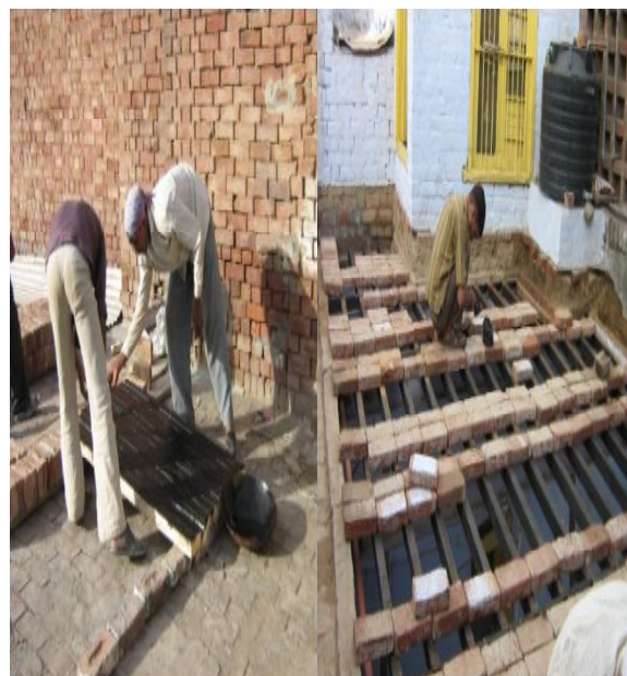
Anti-Termite treatment of purlins
