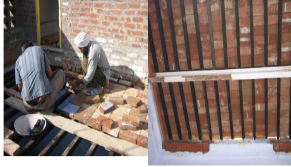
First layer of tile laid
