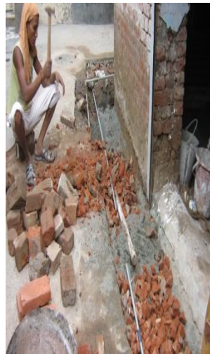
Sand and brick bat layer in plinth protection
