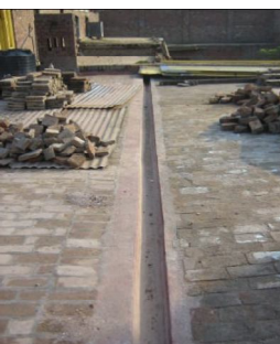
Finished drainage at terrace
