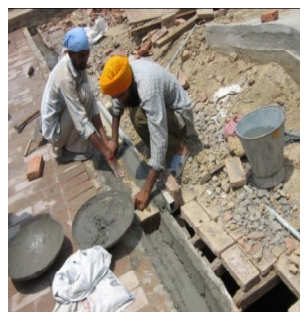
Casting of drainage
