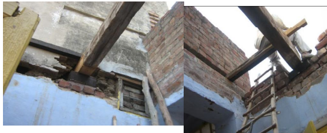
Insertion of wood pad
