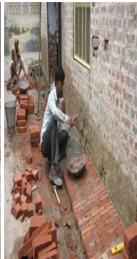
Brick on edge plinth protection in dry lime
