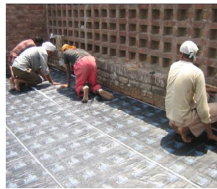
Water proofing layer laid
