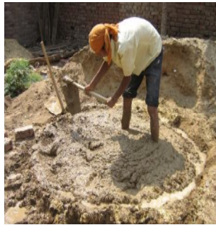
Mud mortar preparation
