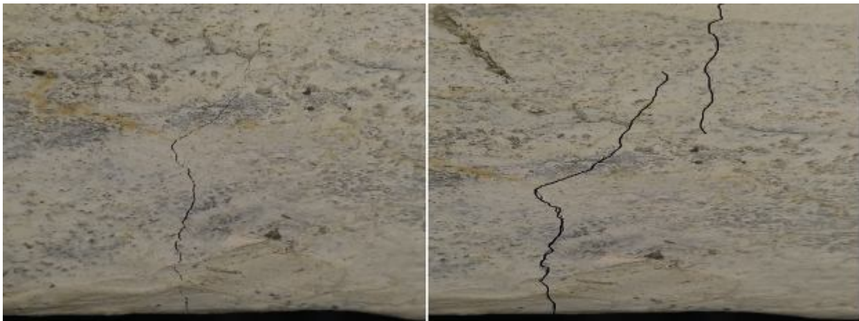
Fig 7: Flexural cracks of the slab specimens
