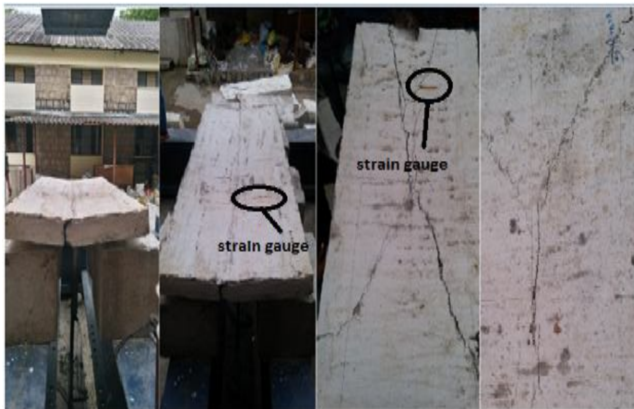
Fig 5: Behaviour of slabs on the compression (top) side
