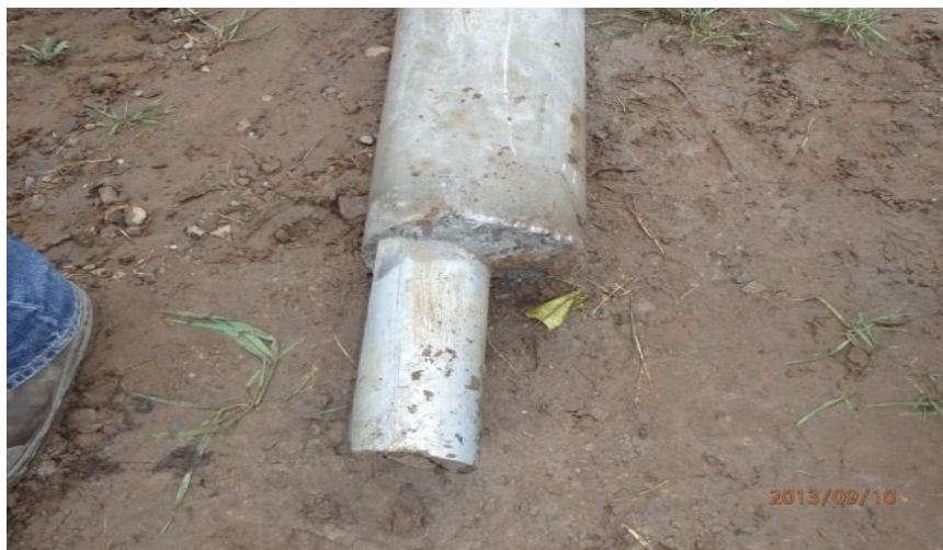
Figure 9. Pile moved into soft soil before concreting
