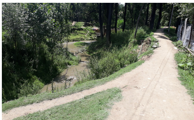
Fig.1: Existing embankment along the bank of river.
