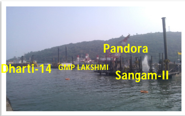
Fig 4.6 Dredging & Drilling/Blasting is in progress Block-F
