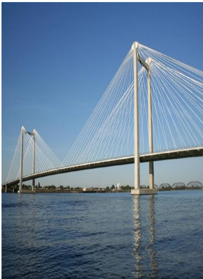
Fig-2: Cable stayed Bridge
