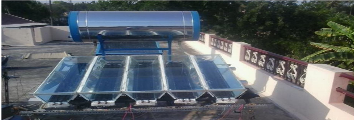
Fig no: 7 Construction of v-trough
