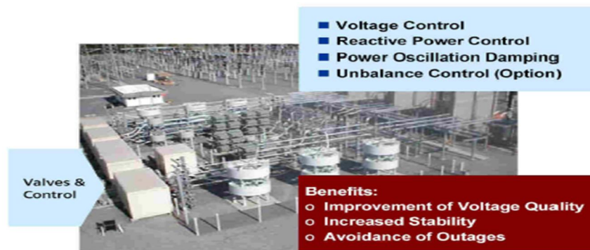
Fig. 6: SVC – Site View and Control Functions
