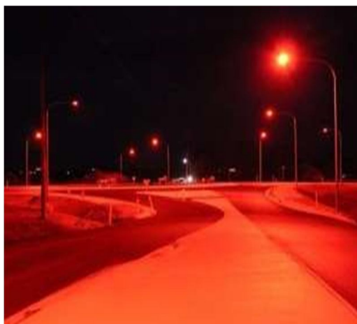
(c) Street lights turned red and alarms switched
