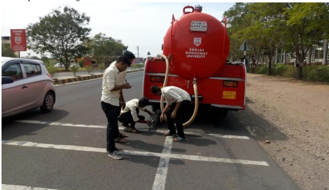
Fig.2 Benkelman Beam Deflection measurement to collect pavement data
