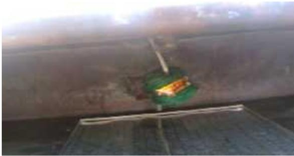
Fig.7 positioning the explosive
