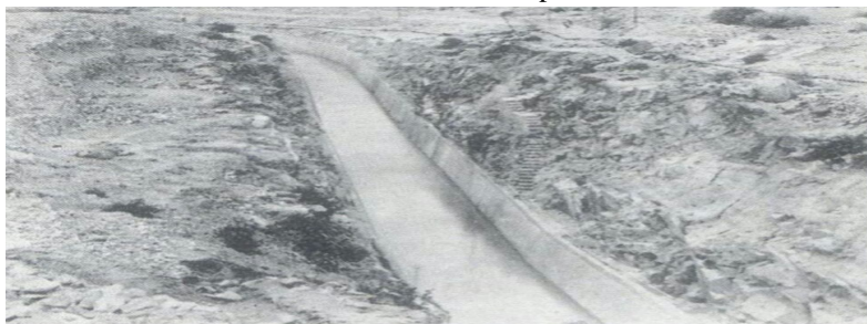
Fig 2. Cement Concrete Canal Lining
