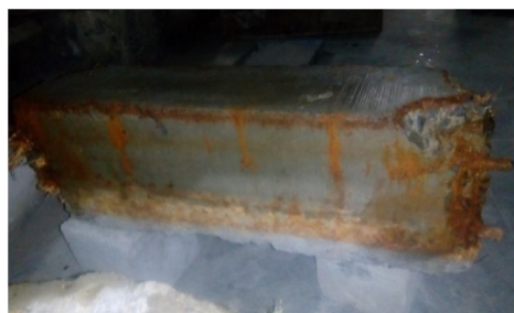
Fig.7 Corroded beam.
