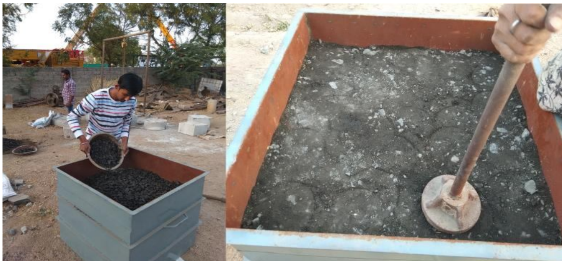
Figure 8 Laying and Compaction of Base course/WMM
