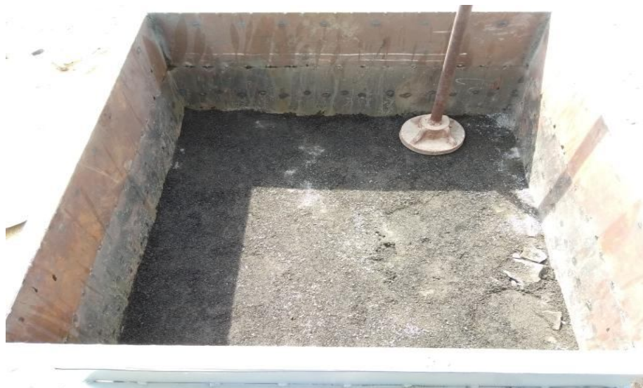
Figure 6 Laying and Compaction of WBM
