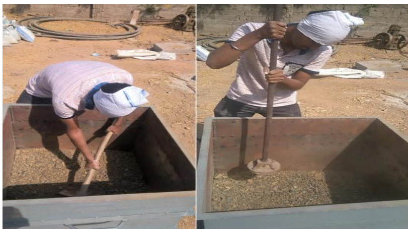
Figure 4 Laying and Compaction of Subgrade
