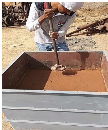
Figure 7 Laying and Compaction of WBM final layer
