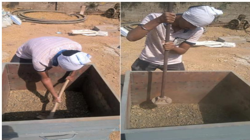
Figure 4 Laying and Compaction of Subgrade
