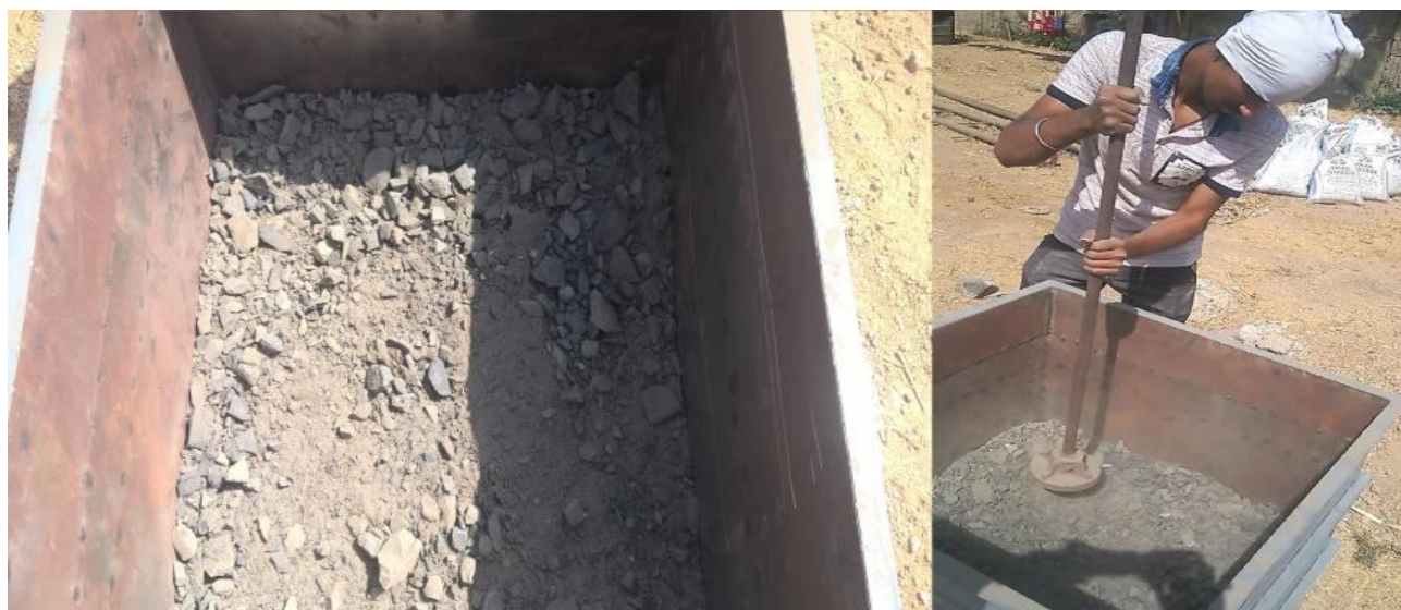
Figure 5 Laying and Compaction of Subbase
