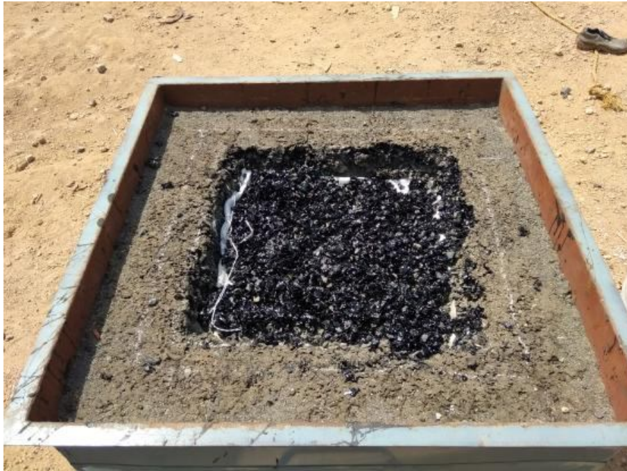
Figure 15 Laying of Bitumen Concrete
