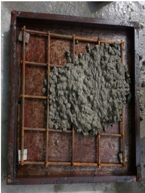
Figure 2: Slab mould with reinforcement
