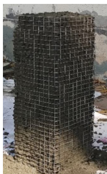
Fig. 2 ferrocement jacketing
