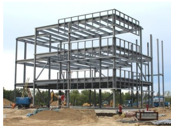
Fig. 2: Steel Frame structure
