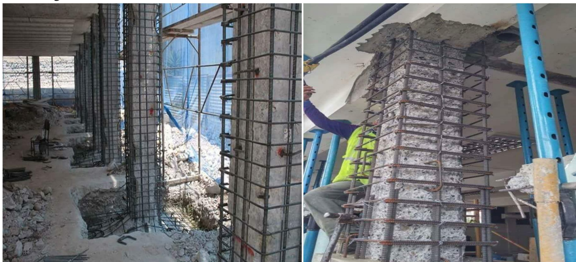
Fig. 8 Retrofitting in Columns by Concrete Jacketing
