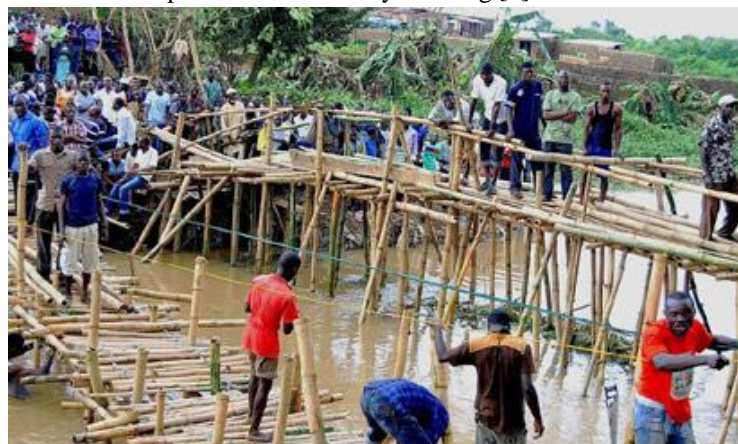
Fig. 2: showing Apete Pedestal Bridge under construction
