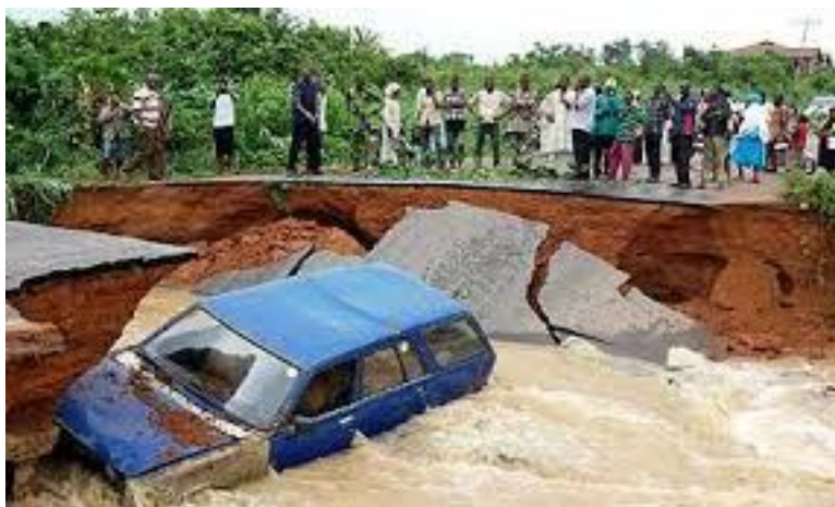
Fig. 1: showing Apete River Flood in action.
