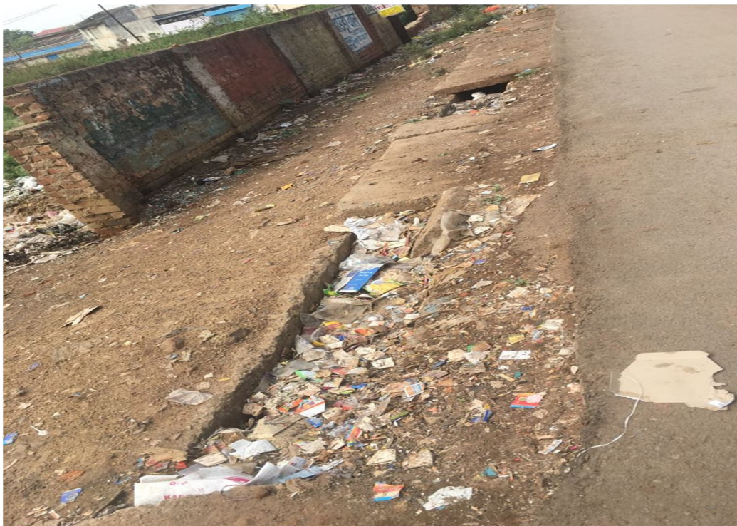
Fig.1 Gudhiyari Road Raipur
