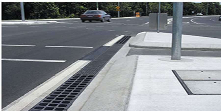
Fig. 4 SLOTTED INLETS
