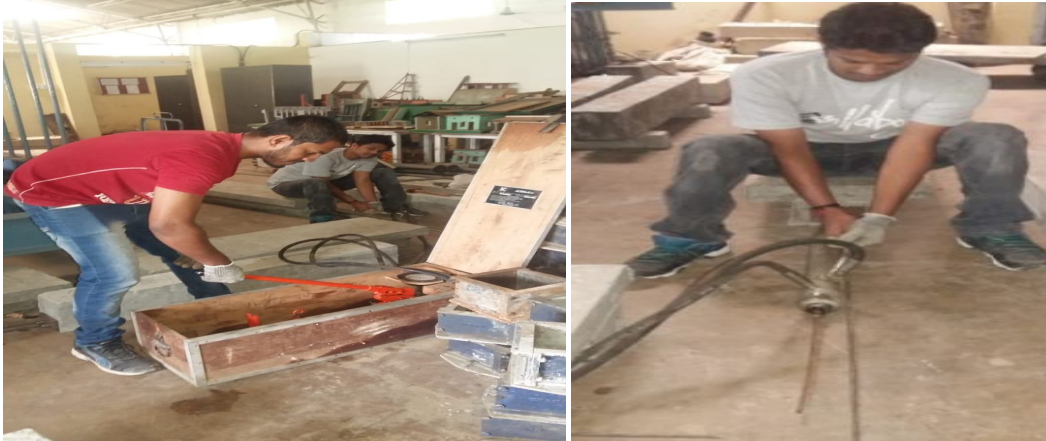
Figure.3. Post-tensioning of beams
